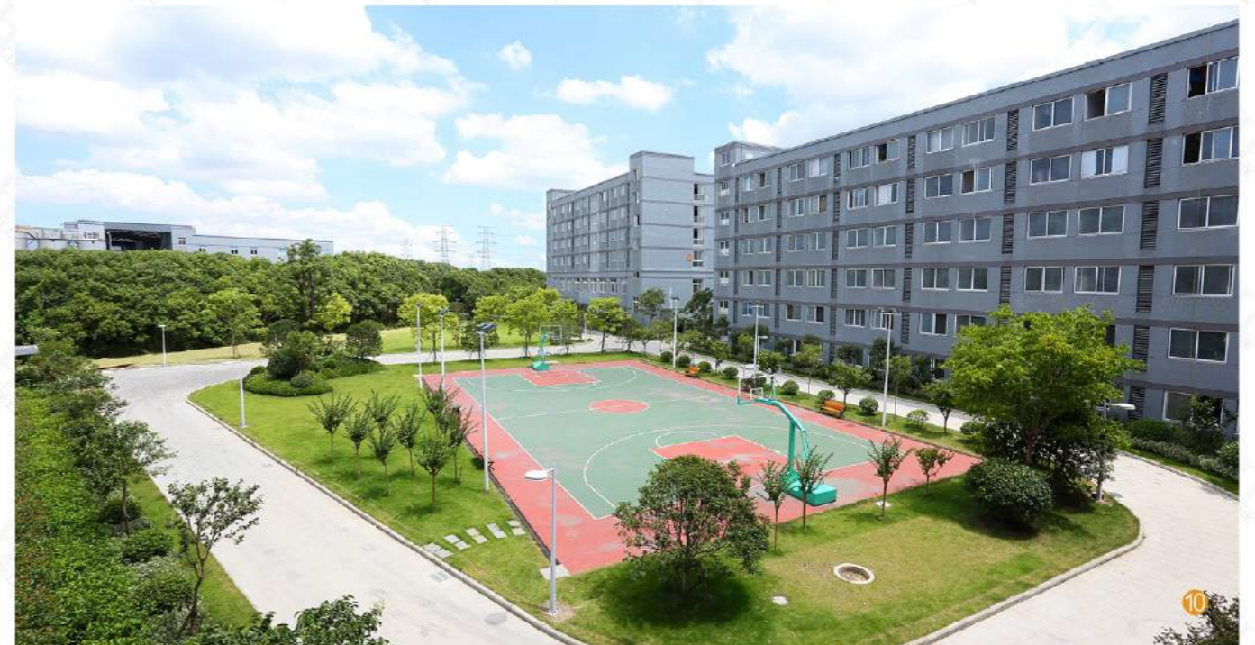
10. Completed new campus
